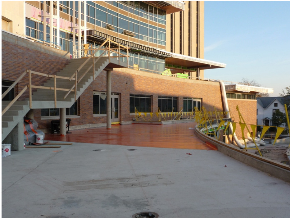
Tour Photo: Another view of the terrace under construction.
